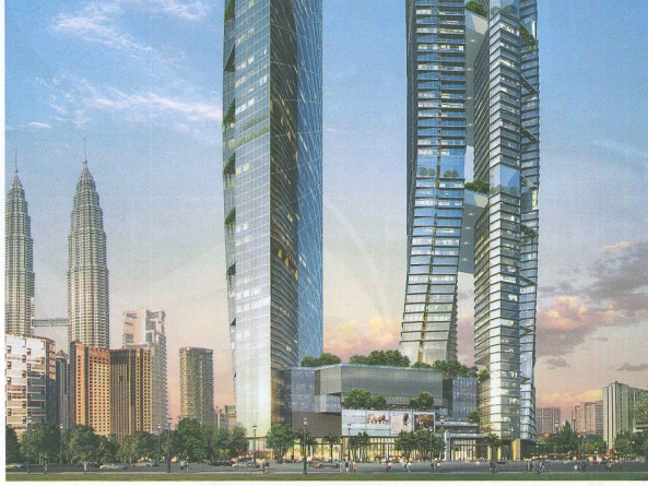
8 Conlay, which has a GDV of RM5.4 billion, features interior designs by Kelly Hoppen (Tower B) and Steve Leung (Tower A)
